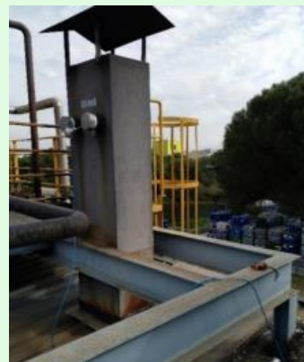
Figure 12: chimney for WHRU installation
