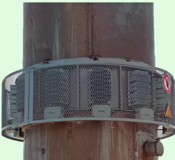
Figure 5: installed WHRUs
